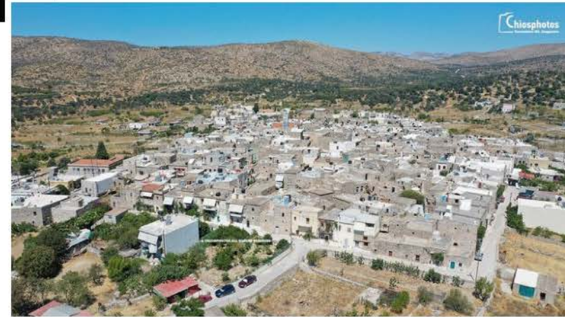
□ Medieval Mastic Village of Olympoi, Chios, Greece.
